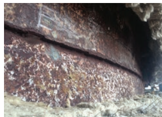
Skirt-to-shell cracking
