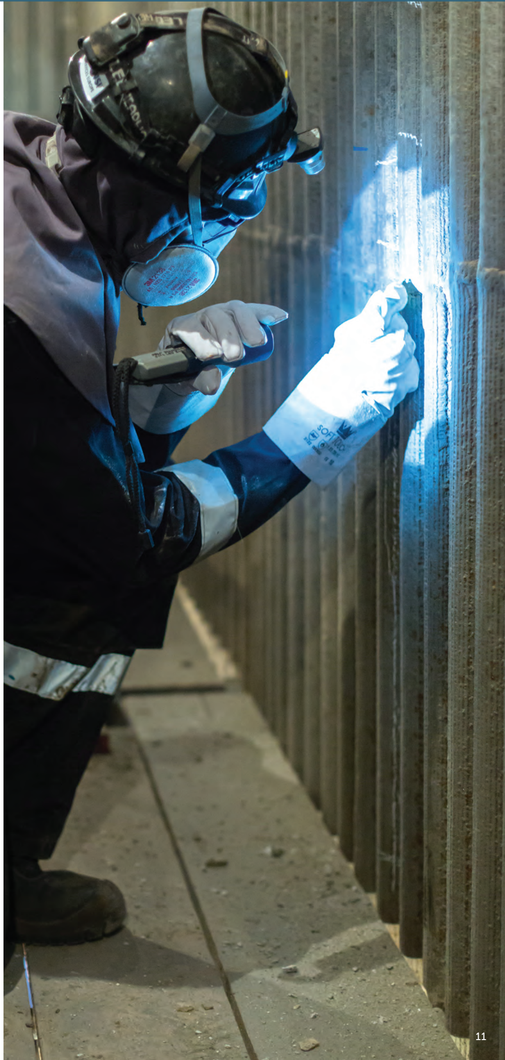
Field inspection of existing overlay
