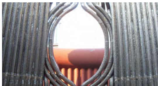
Spiral tubes with windows
