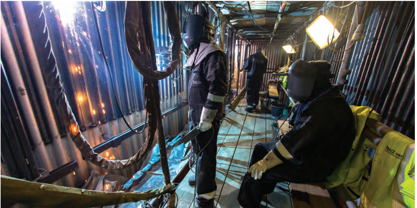
Waterwall repair at an Energy from Waste facility
